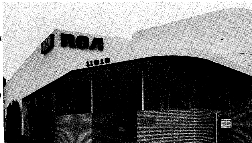
Fig. 2—Aviation Equipment Department, West Los Angeles.
